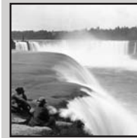
UNITED STATES ADAMS POWERHOUSE AT NIAGARA FALLS
