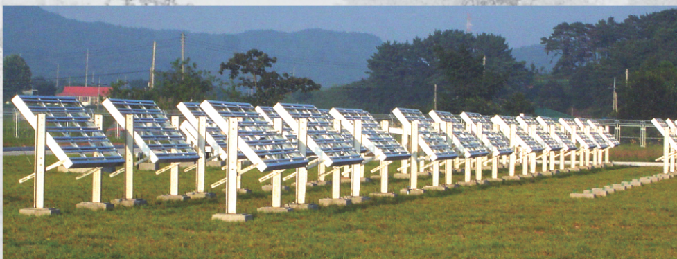
Direct Exposure Rack
