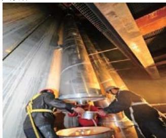
Cable installation requires more professional commissioning team; the installation cost is much higher than AZZ GIL; and the installation of vertical and inclined shafts is more complicate. 电缆安装需要专业的安装队伍, 安装成本远高于AZZ GIL, 竖井和斜井的安装更为困难
