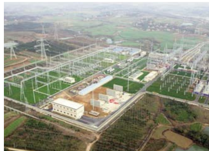
Airscape view of Jingmen Substation
