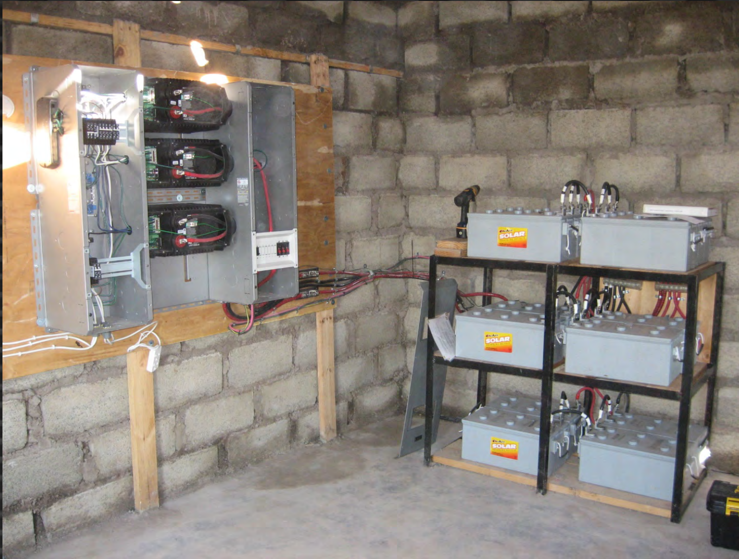
One of Five Systems installed in 2008 in N'Kau Lesotho Africa Three 3.0 kW Inverter/Chargers - 9.0 kW Total 230/400 VAC Three Phase
