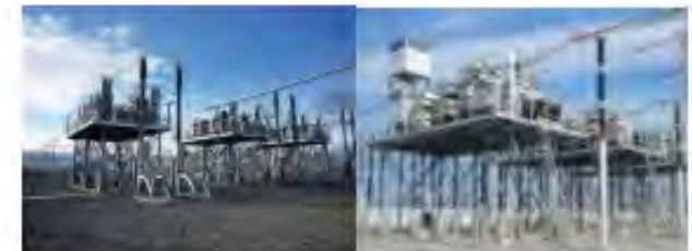
Fixed Series Compensation (FSC)
