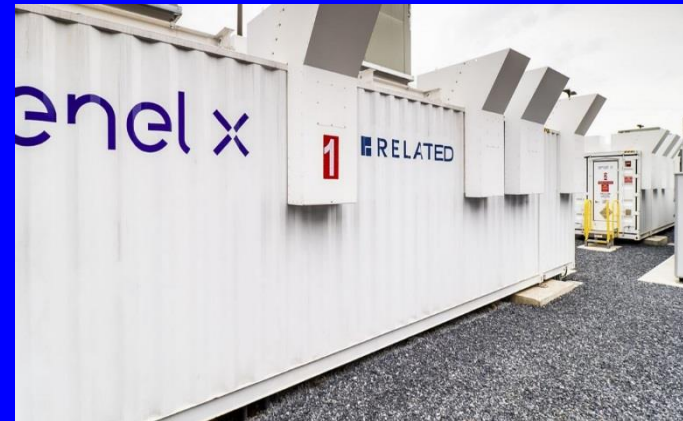
Li-ion batteries by ENEL-X
