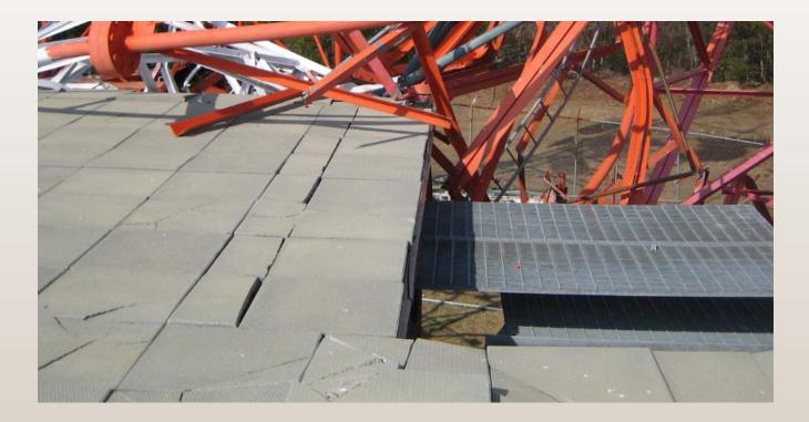
Coordination of Design Disciplines (Arch & Struct) Wind Uplift on deck w/MASP: line load ≠ uniform load
